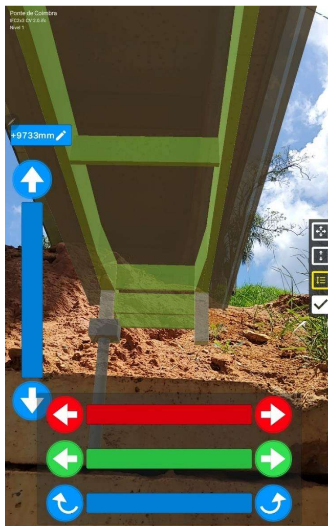
Figure 9. Positioning the BIM model on the physical structure.
