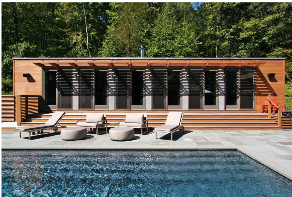
Figura 35: Fachada Connecticut Pool House
