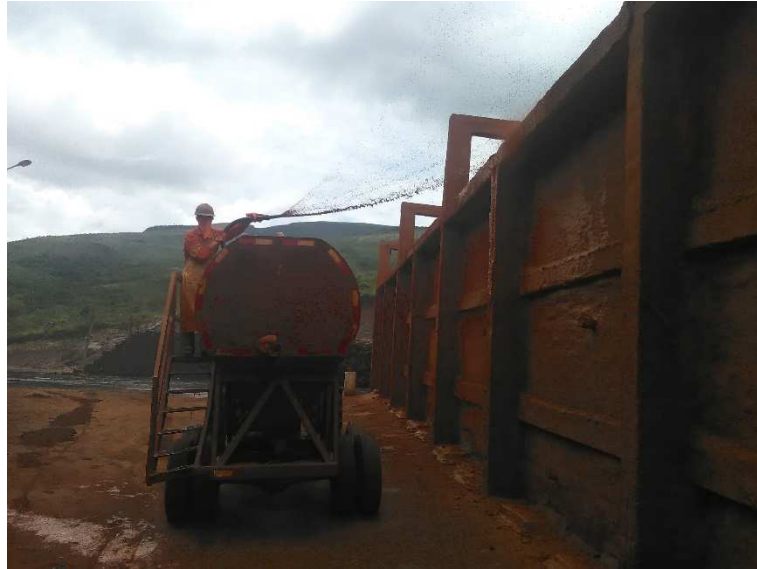
Figure2. Application of mortar over the carbonization kiln in the cooling stage. PAM Bioenergy (2016).
