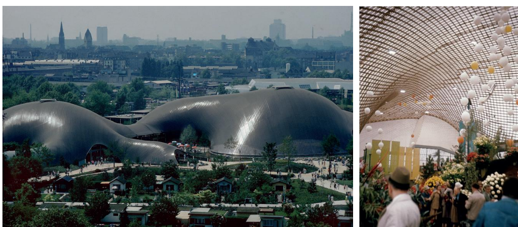
Figura 3 – Cobertura do Multihalle and Restaurant .
