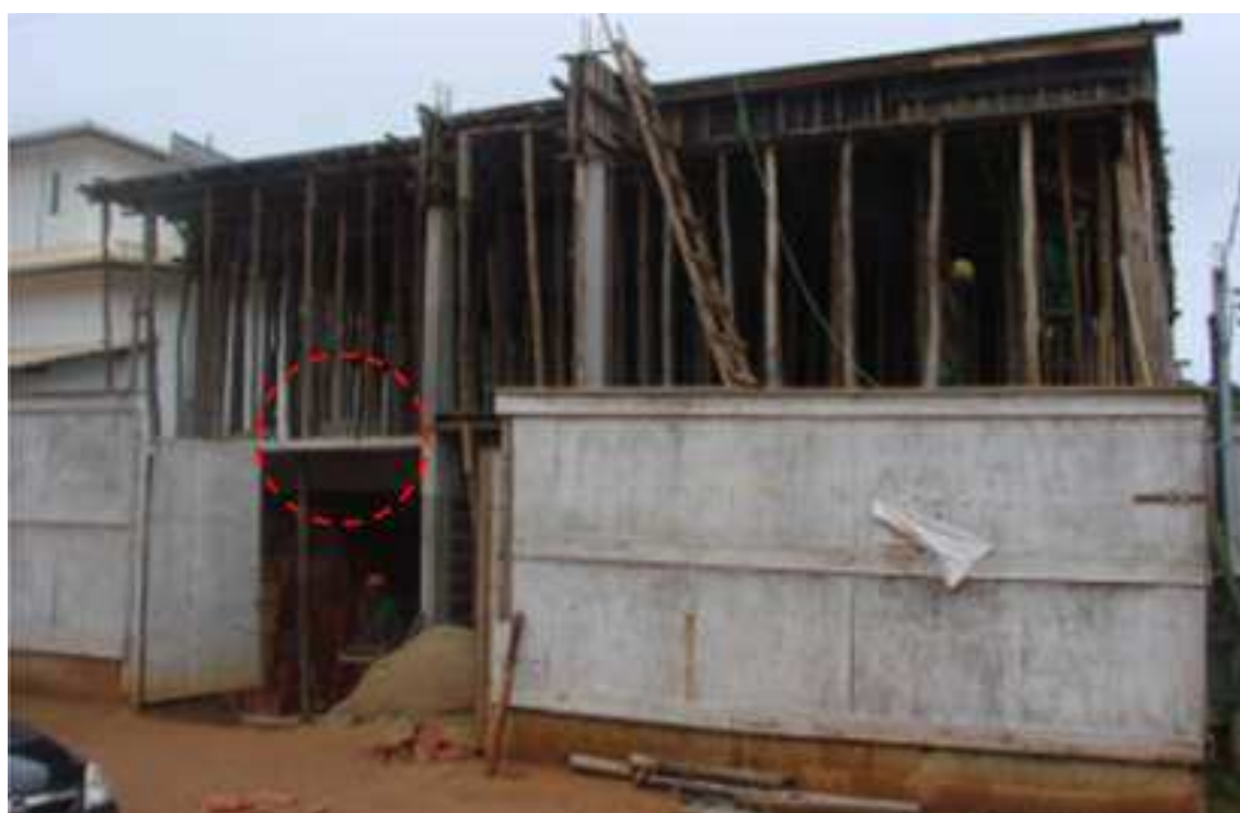
Figura 31 - Obra 2 - concreto com f_{ck} = 25,0 MPa.
