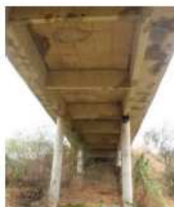
Figure 8. Lower view of Peixe River Bridge.
