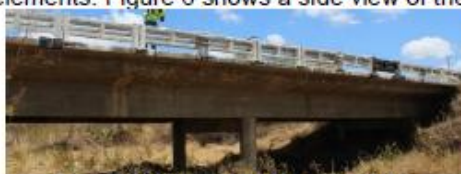
Figure 6. Side view of Latadinha Brook Bridge.
