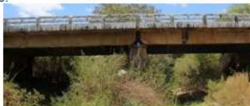
Figure 1. Side view of Zé Dias Brook Bridge.
