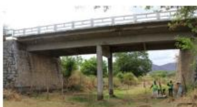
Figure 3. Side view of km 0.91 Bridge.
