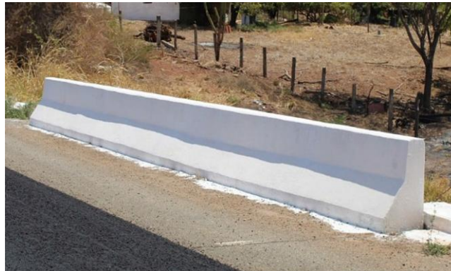
Figure 8 - New Jersey Barrier.
