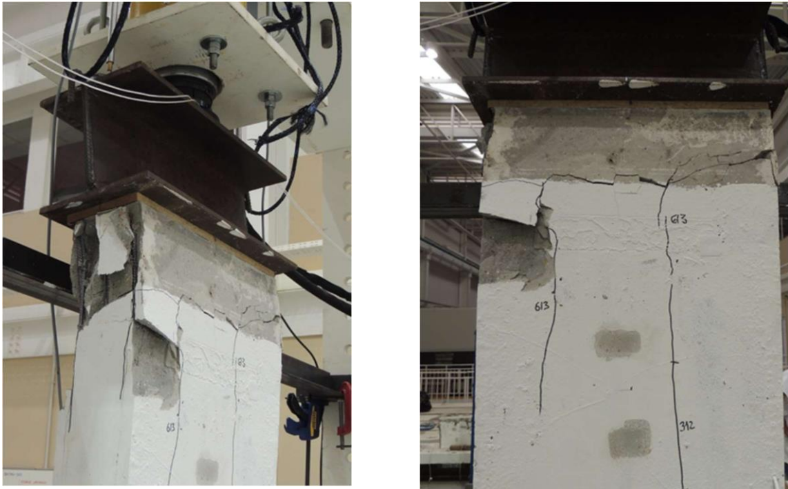
Figure 3.8 - Cracking patterns observed in PA1.
