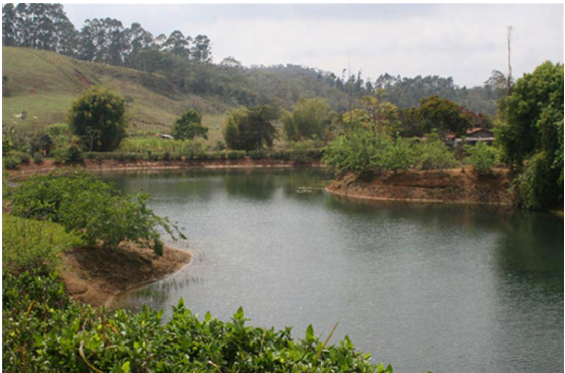
APPENDIX A. Overview of the Sossego Dam at Latão Stream
