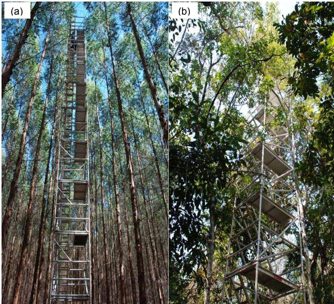
Figure 5. Micrometeorology tower at eucalyptus plantations (36 m, a) and Savanna biome (20 m, b) of experimental site in Brazilian Tropics.
