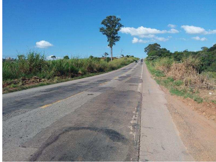
Figure 3: Paved road situated at Alfenas, Minas Gerais (CNT, 2018).
