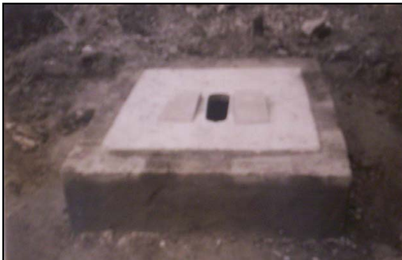
Figura 3.12 – Concrete slaby properly placed. (Laje de concreto)
