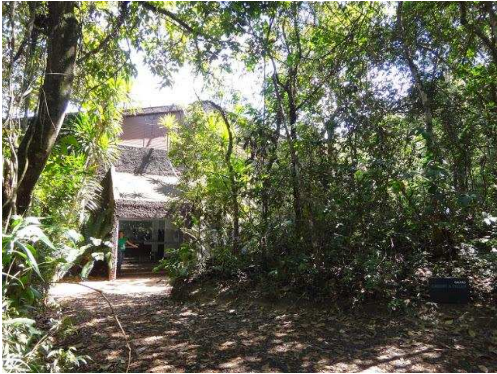
Image 5.9 Galpão Cardiff&Miller, site photo, entrance door Source: <artigoedefinido.com.br>
