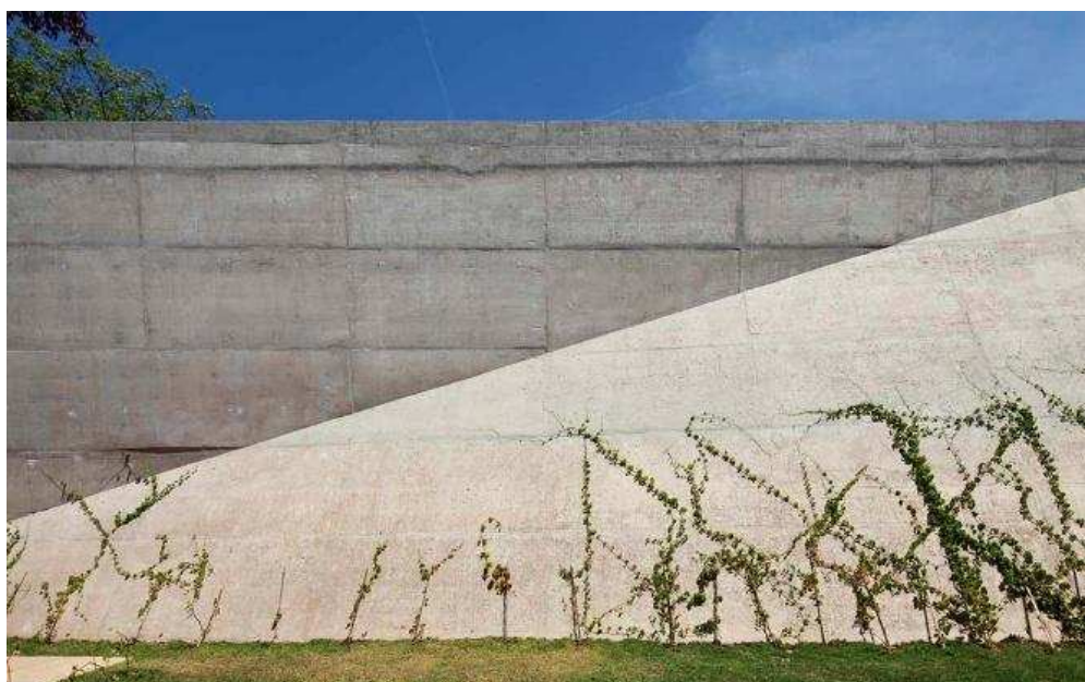
Image 4.11 Galeria Lygia Pape by Rizoma Arquitetura, Façade triangulation Source: <cargocollective.com>
