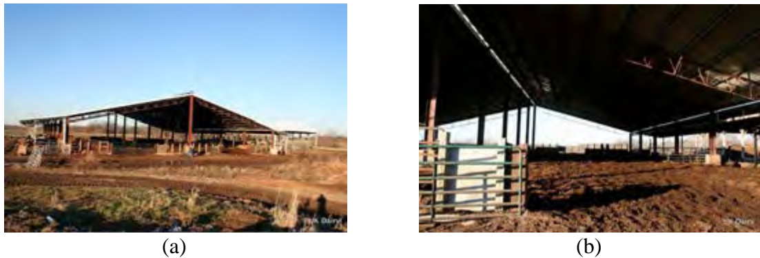
Figure 4.35 - The main constructive characteristic of CBP barn 31.
