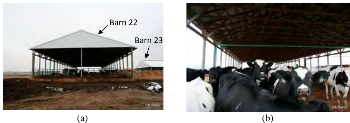
Figure 4.26 - The main constructive characteristic of CBP barn 22.
