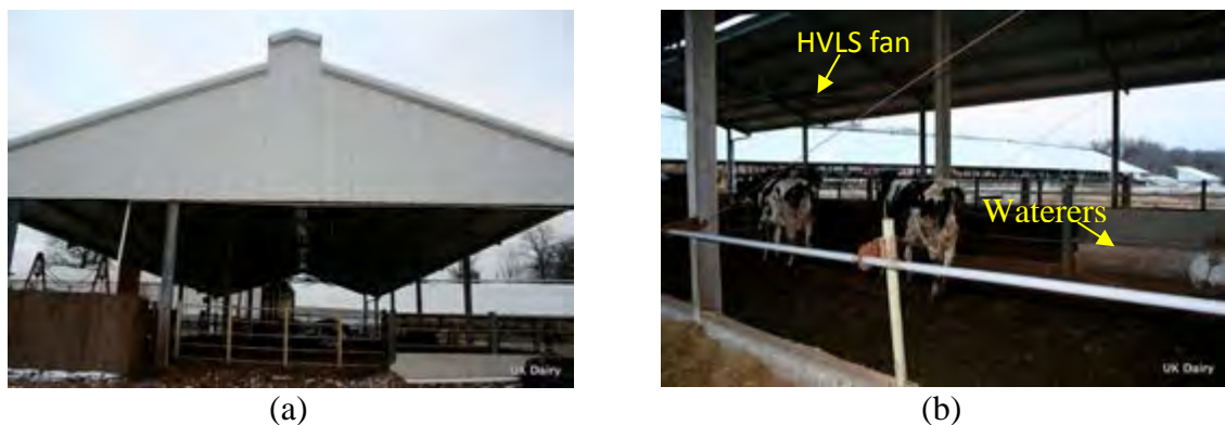
Figure 4.39 - The main constructive characteristic of CBP barn 35.
