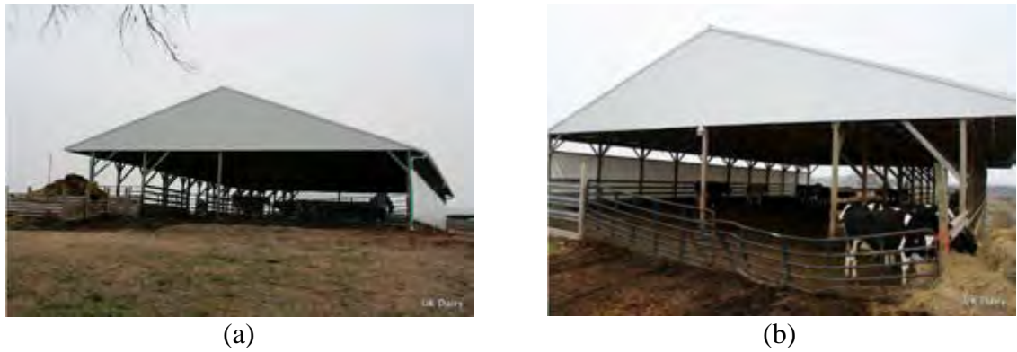
Figure 4.28 - The main constructive characteristic of CBP barn 24.
