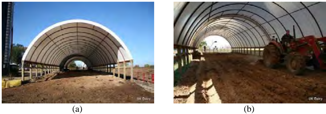
Figure 4.10 - The main constructive characteristic of CBP barn 4.
