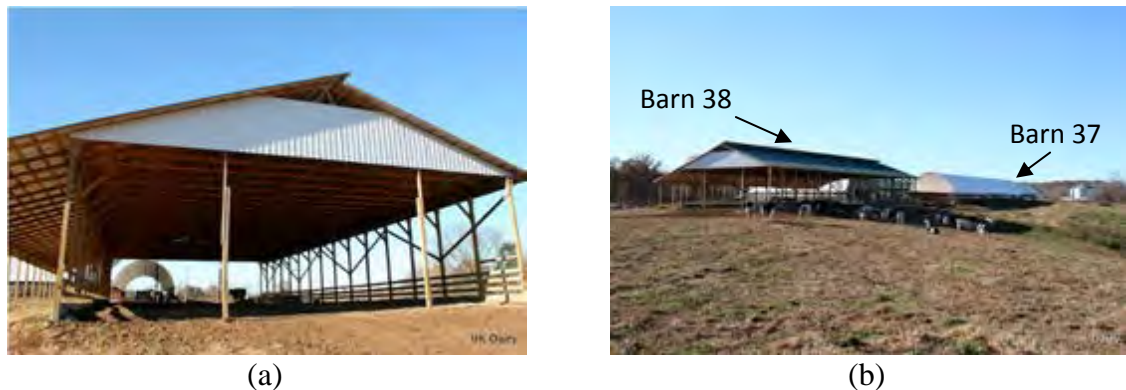
Figure 4.42 - The main constructive characteristic of Barn 38.
