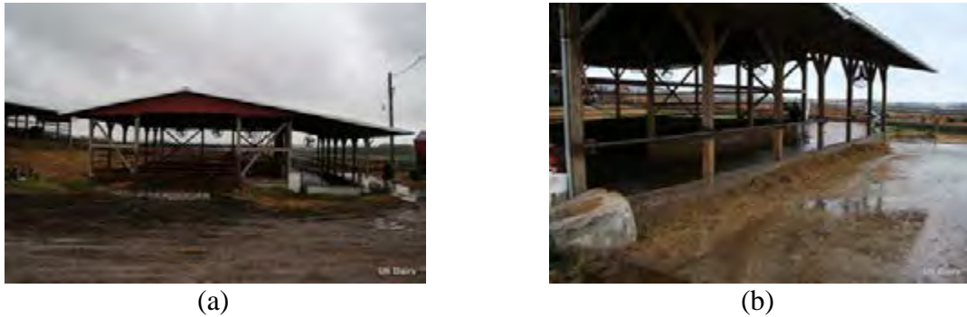
Figure 4.20 - The main constructive characteristic of CBP barn 16.
