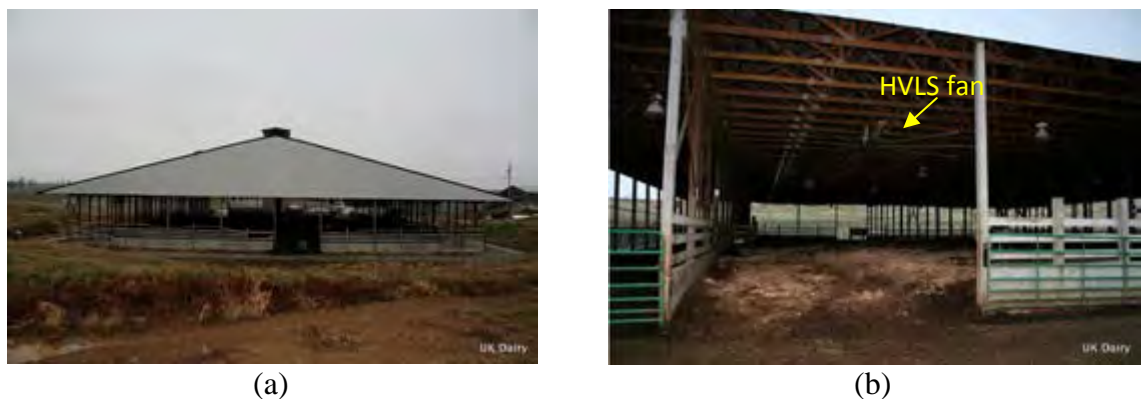
Figure 4.29 - The main constructive characteristic of CBP barn 25.
