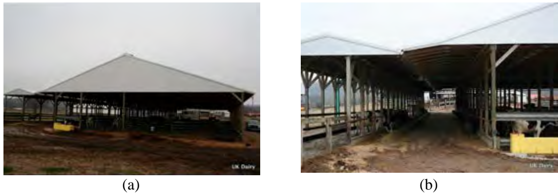
Figure 4.27 - The main constructive characteristic of CPB barn 23.
