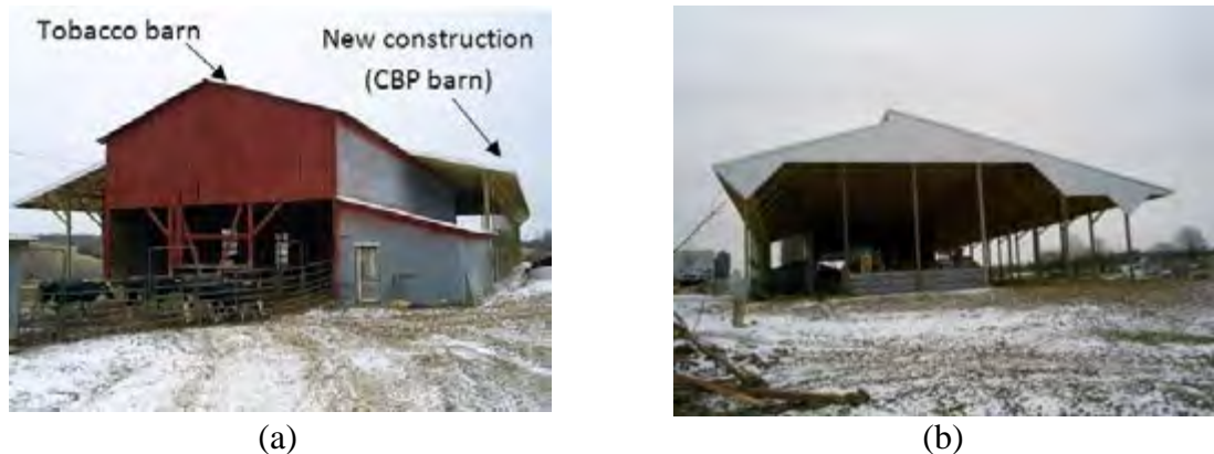
Figure 4.38 - The main constructive characteristic of CPB barn 34.
