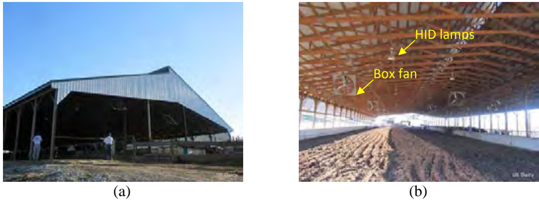
Figure 4.15 - The main constructive characteristic of CBP barn 9.
