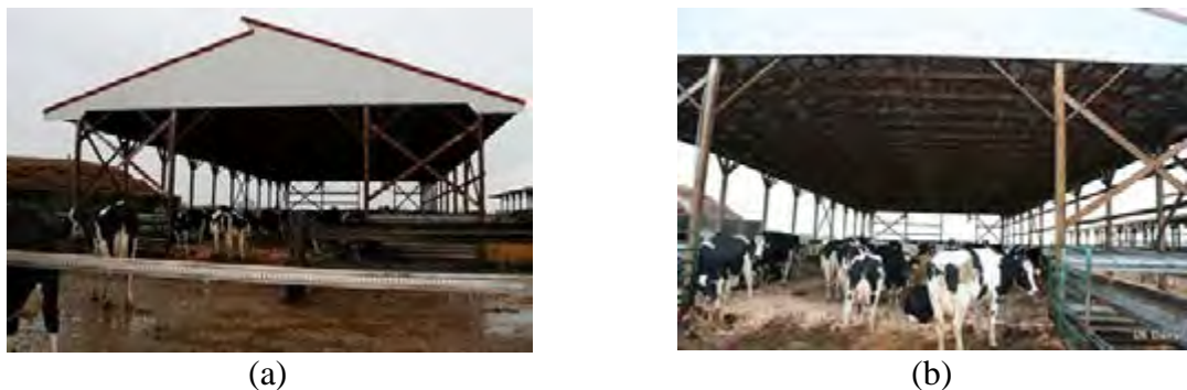
Figure 4.21 - The main constructive characteristic of CBP barn 17.
